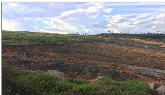
Gambar 4. Area longsor floor 3000
